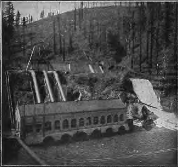
FIG. 105.—Modern hydro-electric power plant, Cazadero, Oregon. Cement dam, steel tube penstocks. Type of construction for high fall. (From Power Development by F. Koester.)
